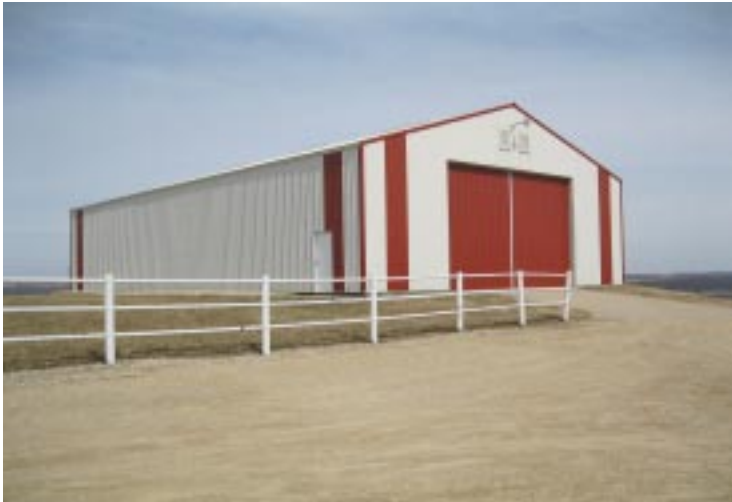
80' x 48 Pole Shed-Built in 2001
